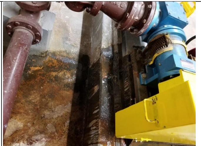
Pump, sludge pump 1 (Score: 5-Very Poor)
