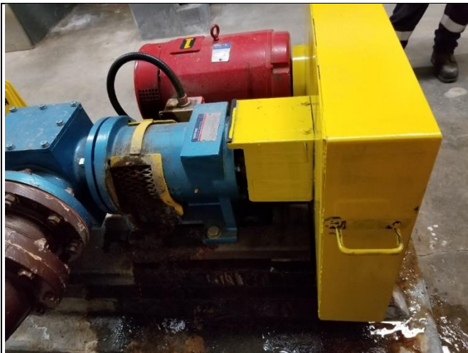
Pump, sludge pump 1 (Score: 5-Very Poor)
